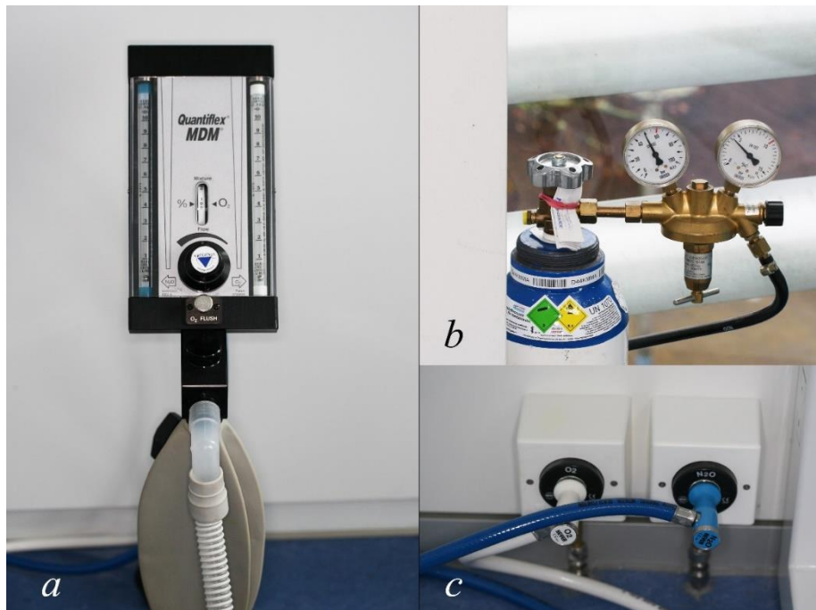
Figure 1: Titratable nitrous oxide system: Quantiflex MDM (a), rental cylinder for nitrous oxide and oxygen (b) and central system for nitrous oxide and oxygen (c)
