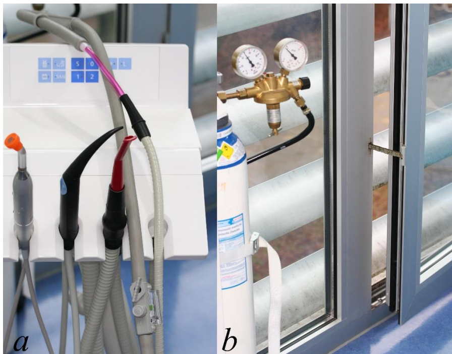
Figure 3: External suction for exhaled air to reduce workplace pollution by nitrous oxide is possible, for example, via the suction system of the treatment unit (a) and room ventilation in the floor area through a large floor window to reduce workplace pollution. Nitrous oxide is heavier than air and therefore sinks to the ground (b)
